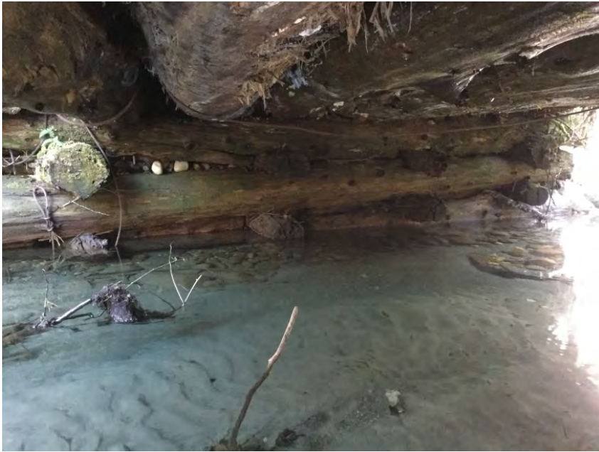
Left Bank Abutment when facing downstream
