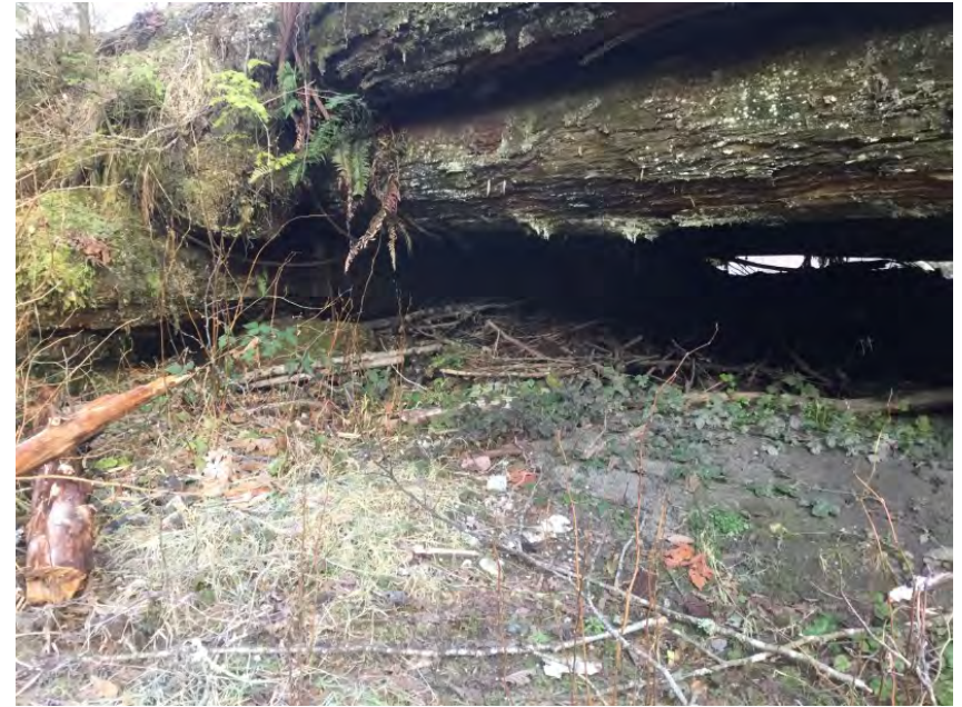
Right Bank Abutment when facing downstream
